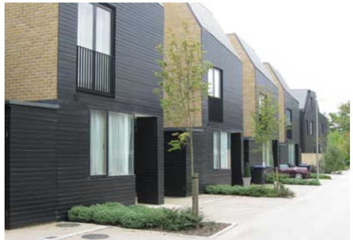
Modern attached building forms can be designed with a degree of separation
