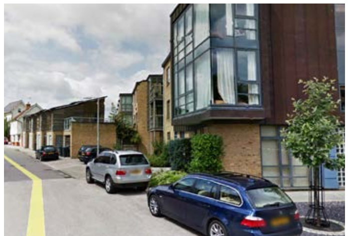
Apartment building with corner window detail
