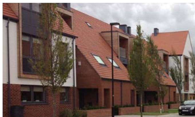
Sloped roof to ground floor emphasises entrances and adds interest
