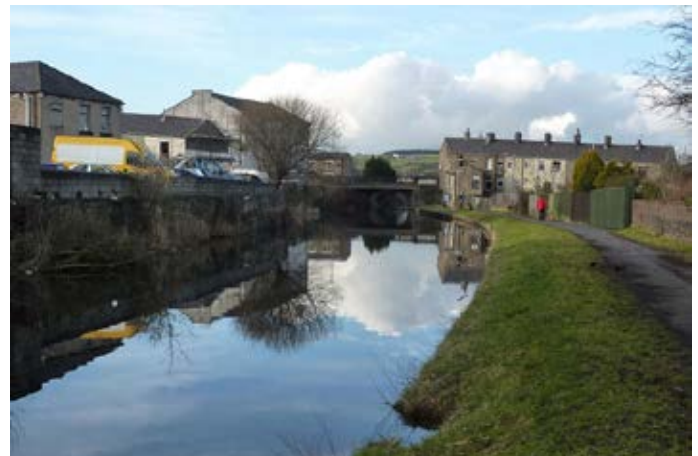
View north to Hermitage Street Bridge
