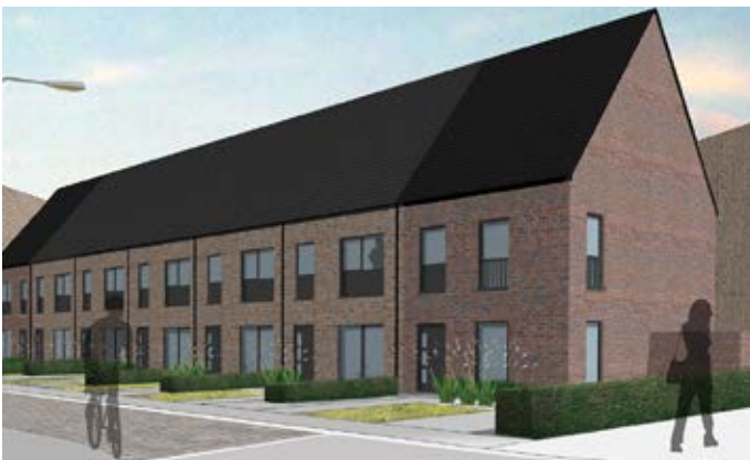
Example of modern terraced housing where detailing is crucial
